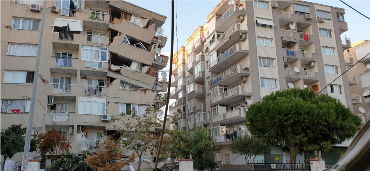
Figure 5.5 Damage observed in the buildings with heavy overhangs.
