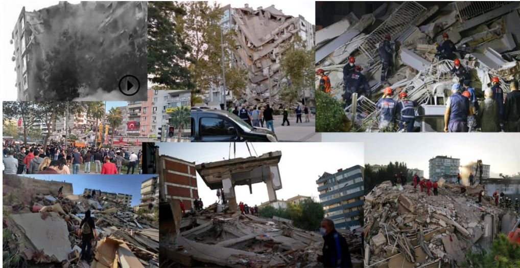
Figure 17. Structural damage in Izmir due to the mainshock (from various sources in the web).
