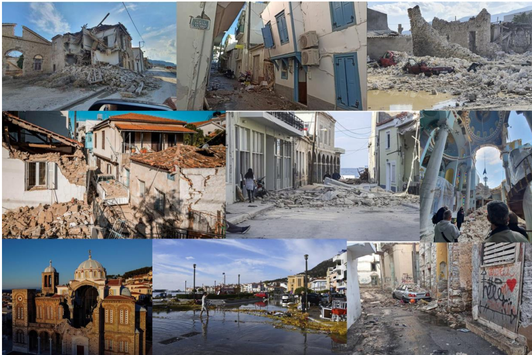
Figure 16. Structural damage in Samos (Vathy) due to the mainshock (from various sources in the web).
