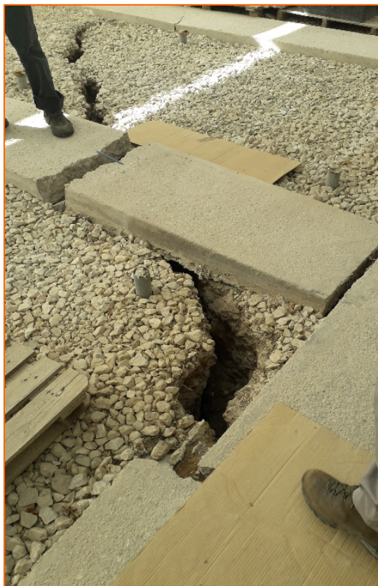
Coseismic surface ruptures and offsets south of Agios Nikolaos village (left) and in the coastal zone of Agios Nikolaos (middle).
