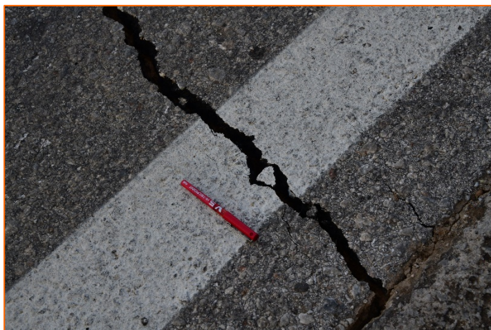
Coseismic surface ruptures observed in the area of Agios Nikolaos
