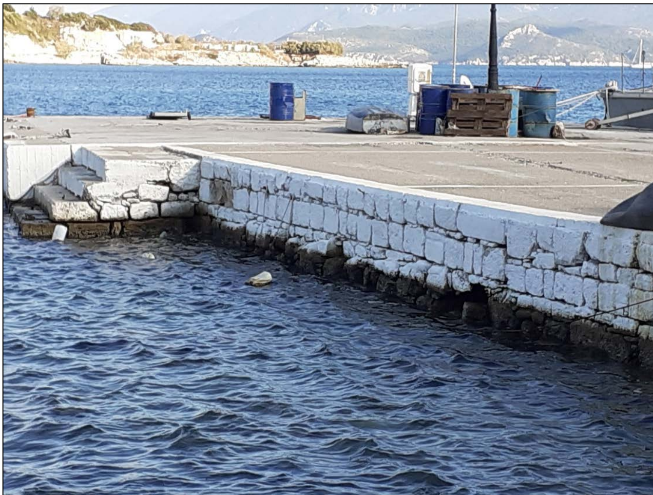
Coseismic uplift of about 20 cm detected in Pythagorio port
