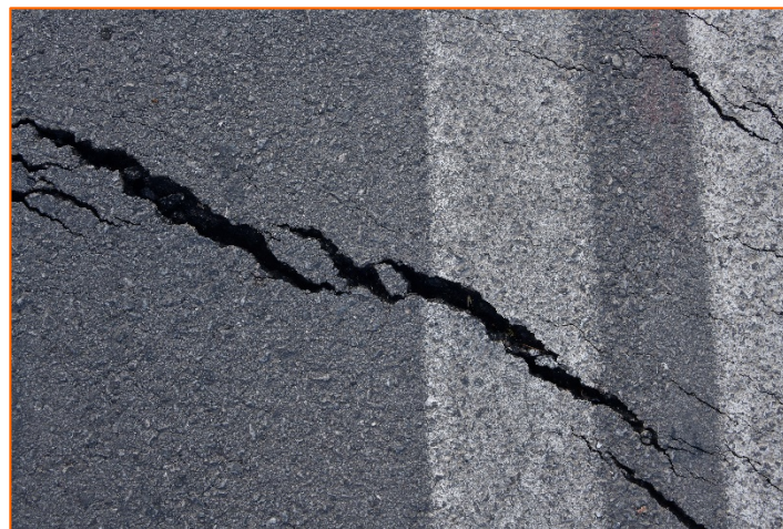
Coseismic surface ruptures observed in the area of Agios Nikolaos
